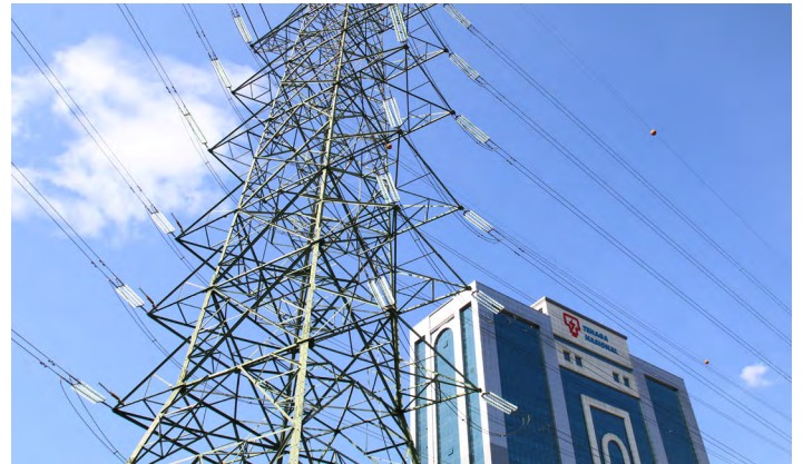
► Tenaga Nasional's transmission tower
